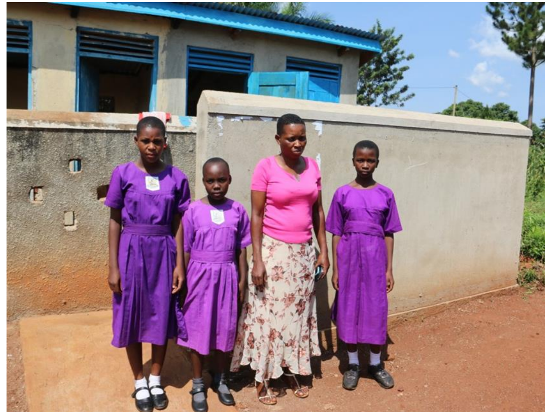
After: Some members of the sanitation committee-Nalinaibi P/S in front of the constructed washrooms
