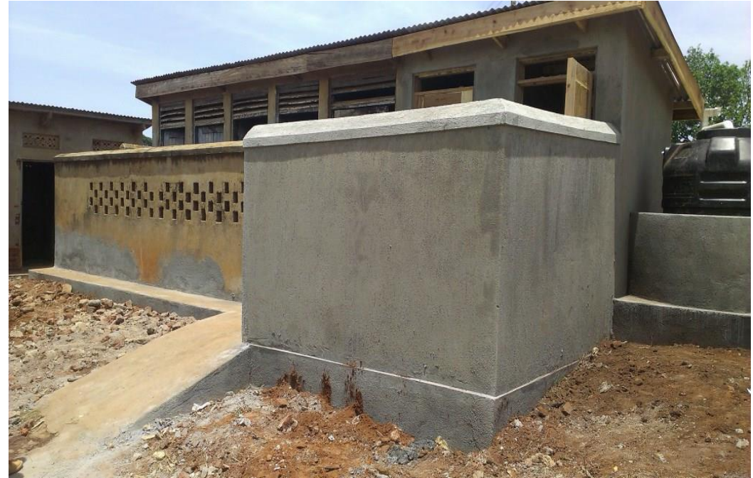
Constructed washrooms in Wabulungu Primary School
